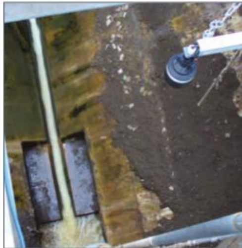
WET WELL 6m WITH LADDER AND FLOAT
