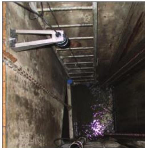
WET WELL 6m WITH LADDER AND FLOAT
