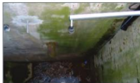
HINGED BRACKET OVER A WET WELL
