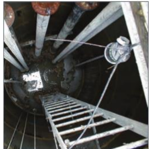
WET WELL 4.5m WITH LADDER AND FAT RING
