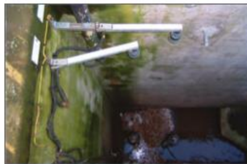
HINGED BRACKET OVER A WET WELL
